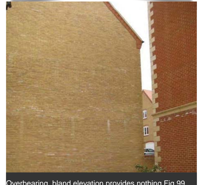
Overbearing, bland elevation provides nothing (Fig 99)
