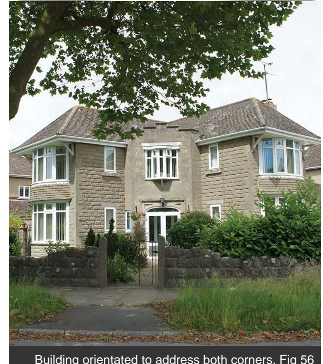
Building orientated to address both corners. Fig 56
