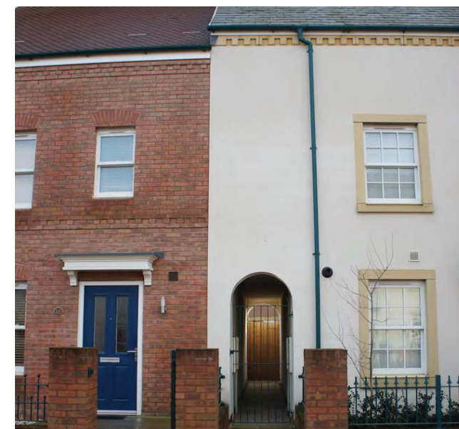
Ginnels provide rear access and storage. Fig 74
