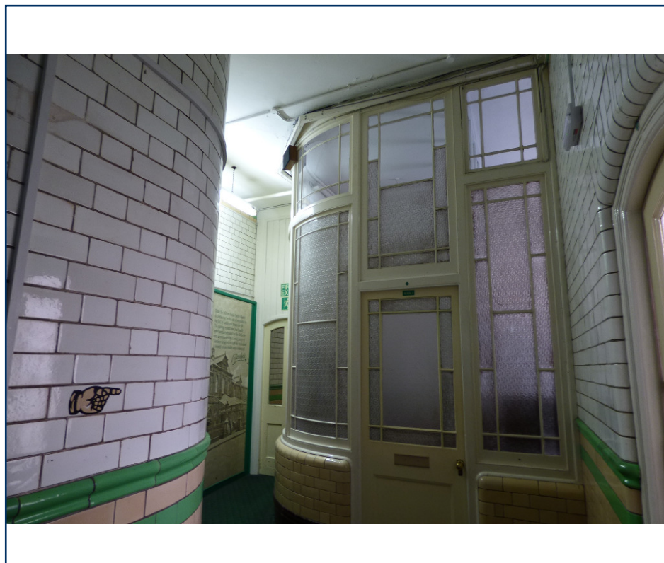
Fig. 26 A fine example of Edwardian construction, including original curved frosted glass. Where would you get that from these days?
