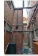
SWHH Central external spine corridor (7)
