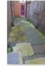
SWHH Central external spine corridor (10)
