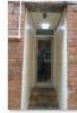
SWHH Central external spine corridor (6)
