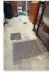
SWHH Central external spine corridor (3)
