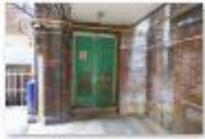
SWHH Central external spine corridor (12)
