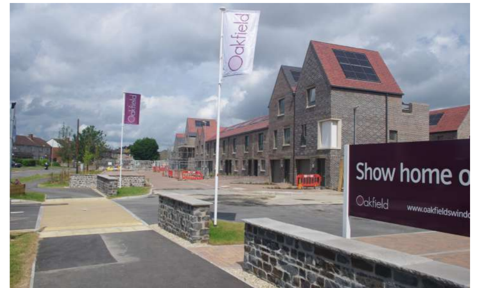
3. Oakfield residential development nearing completion
